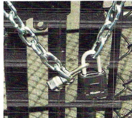
The two locks are daisy-chained. Each lock acts as a link in the chain. Opening either lock unfastens the chain to allow the gate to open.
